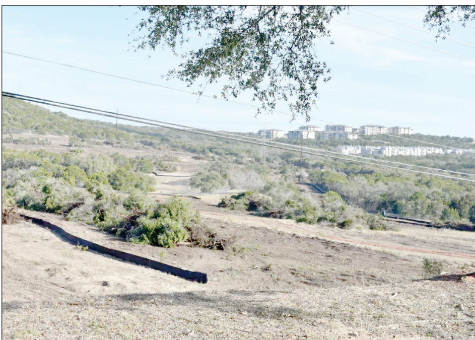
Mixed-Use No. 14, a roughly 80-acre tract on North Quinlan Park Road near the RM 620 entrance to Steiner Ranch, is being developed as a 106 homesite residential project. Leslee Bassman
