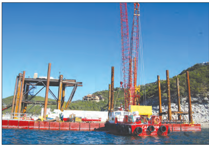
Four Points News staffer joined local media last week for a close-up view of the water intake phase of the City's new Water Treatment Plant #4. The structure is being built about three miles offshore from the system's staging site at Keller Marina.
