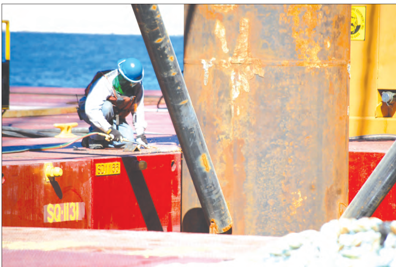
A welder works to construct one of three temporary platforms at the site of WTP4's raw water intake system on Lake Travis.
